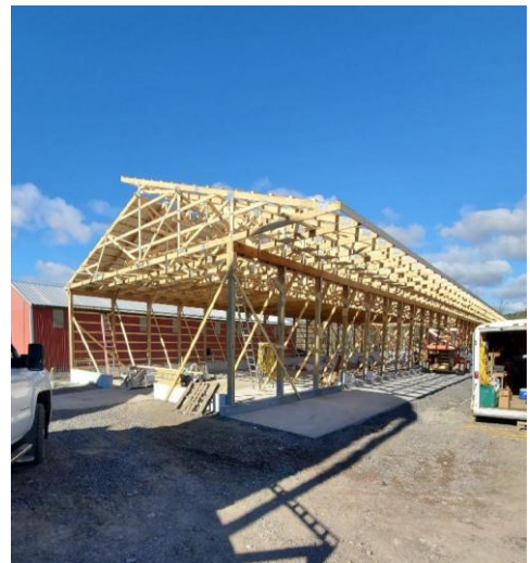
Heavy-use area construction
