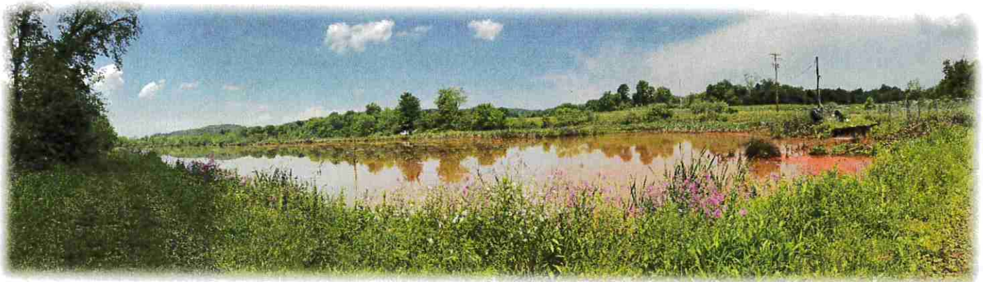
Mine Discharge (right), flowing (left) into the 8 acre treatment system
