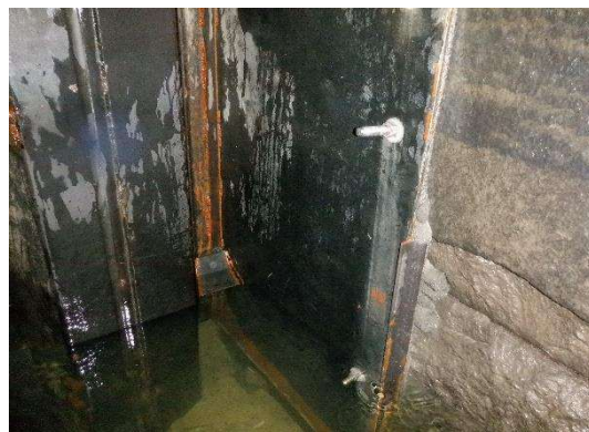
The above photograph shows a sealed gap on the upriver side of the SEPTA Rail Bridge after work was completed.
