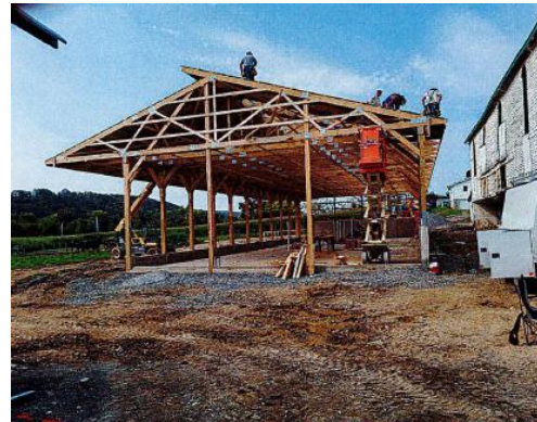
Figure 1: Pfleegor Farm heavy use area construction
