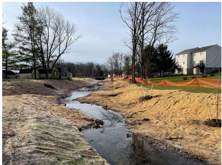
Conoy Creek immediately after restoration
