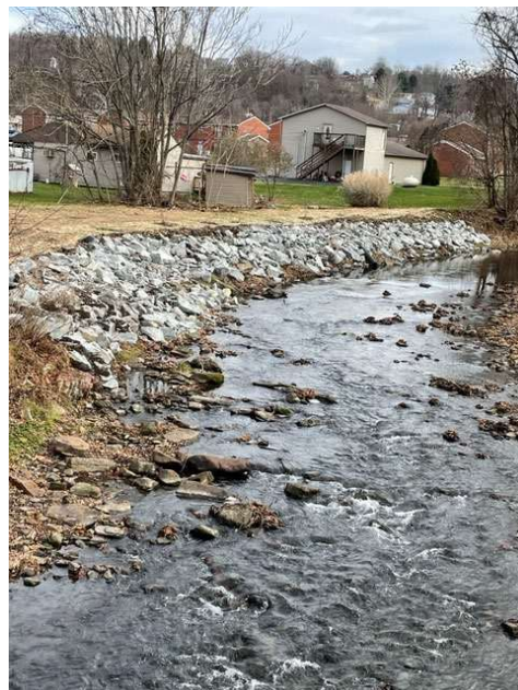
City of Connellsville – Streambank Protection
