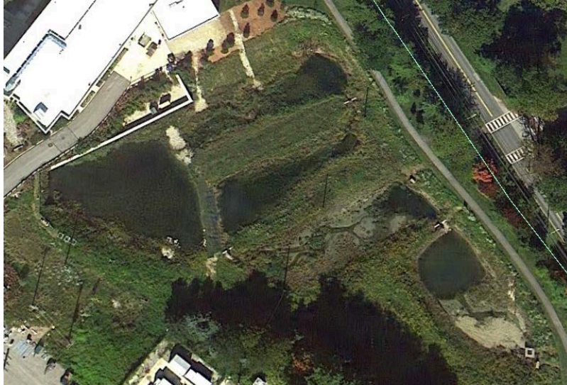
Figure 2 Photograph of VU Constructed Stormwater Wetland from Google Earth (2013).
