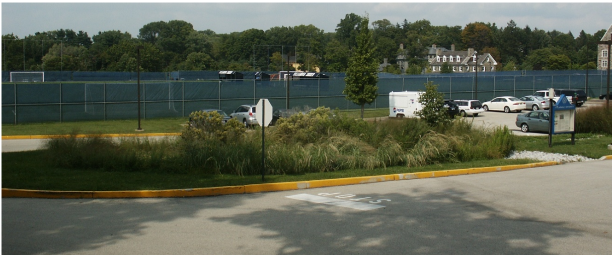
Figure 1. Photograph of VU Bioinfiltration Rain Garden BMP (2007).
