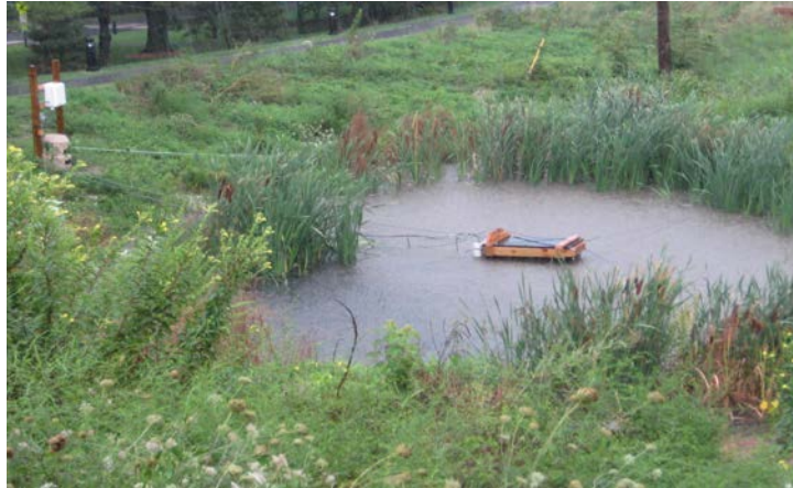
Figure 16. Floating DO instrumentation
