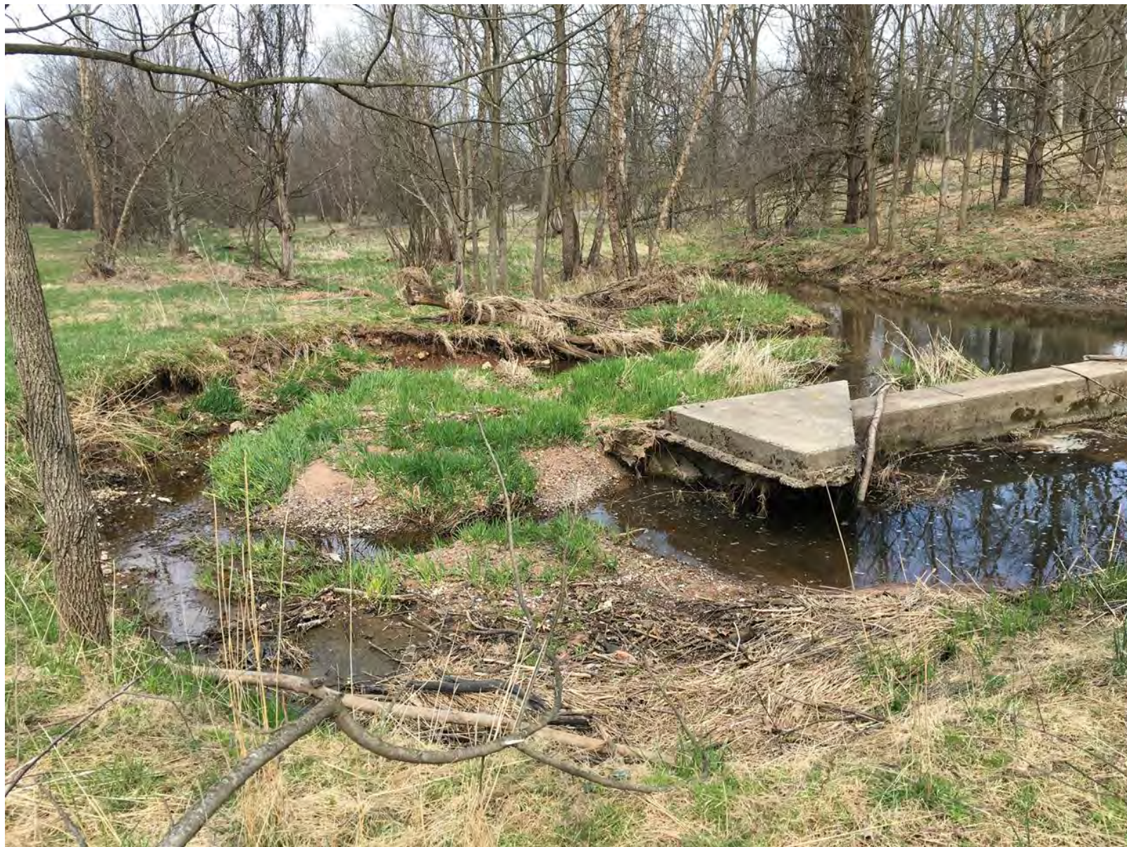
Figure 17. Erosive circumvention of an existing dam in the Spring Creek 319 study area watershed.
