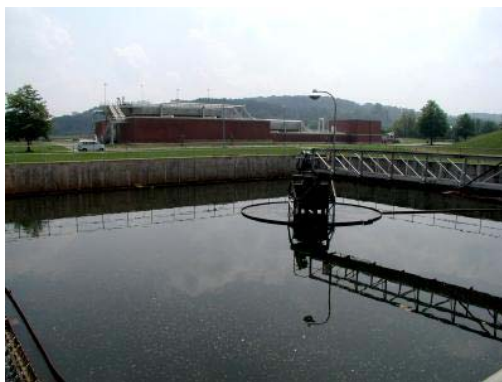
Coagulation Tank – City of Roanoke, VA
