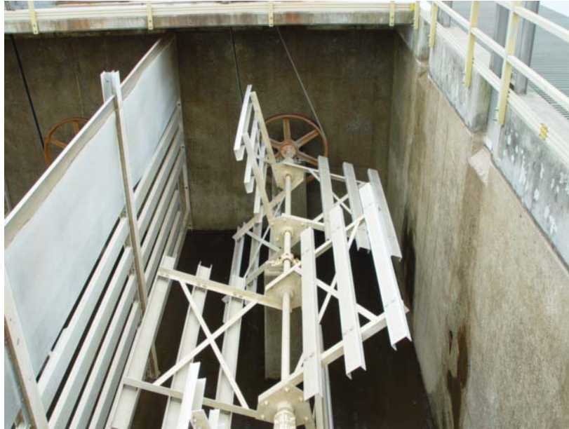
Figure 4.4 – Horizontal Reel Flocculator
