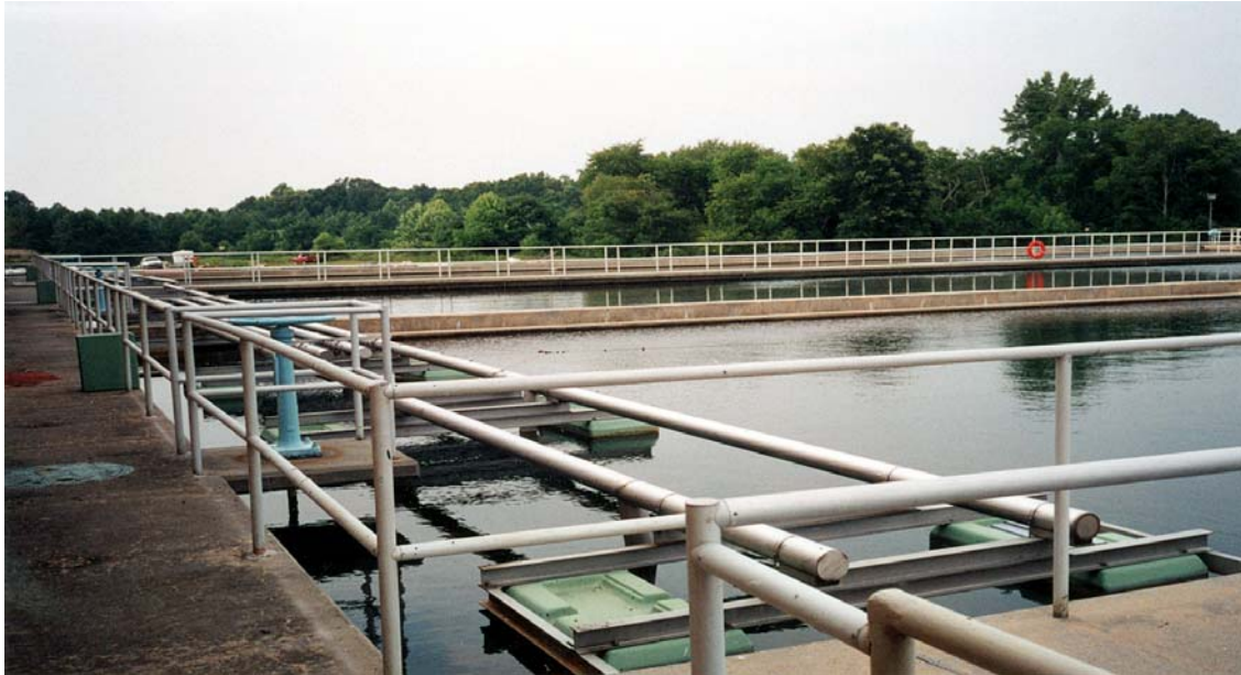
Figure 4.5 – Conventional Sedimentation Basins
