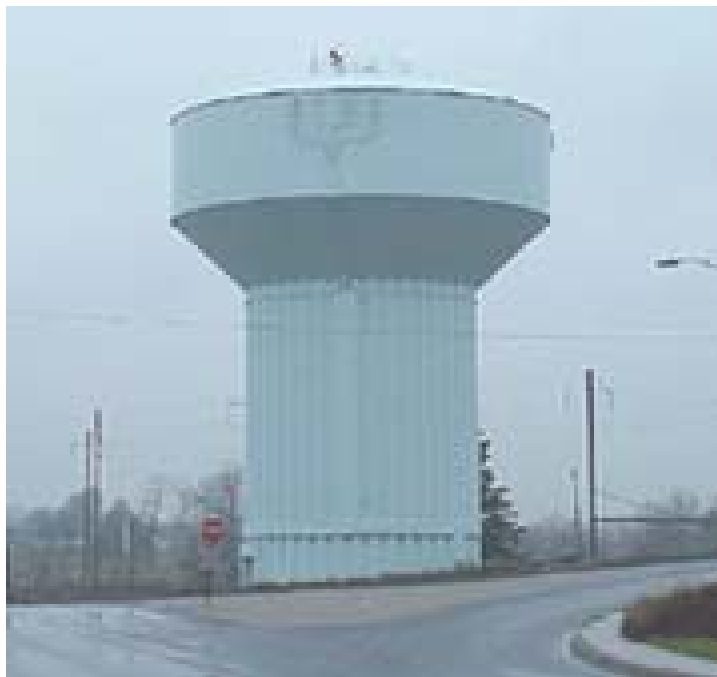
Figure 2.8 – Typical Water Storage Tank in the Distribution System
