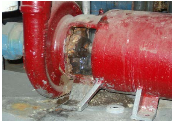
Figure 4.1 Leaking Gland
