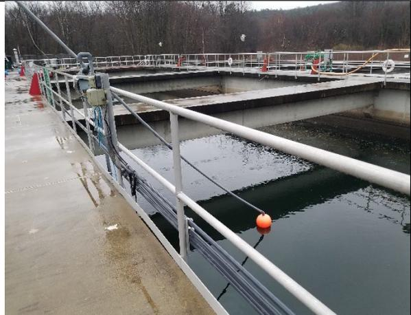
SBR probe float and anchor pole
