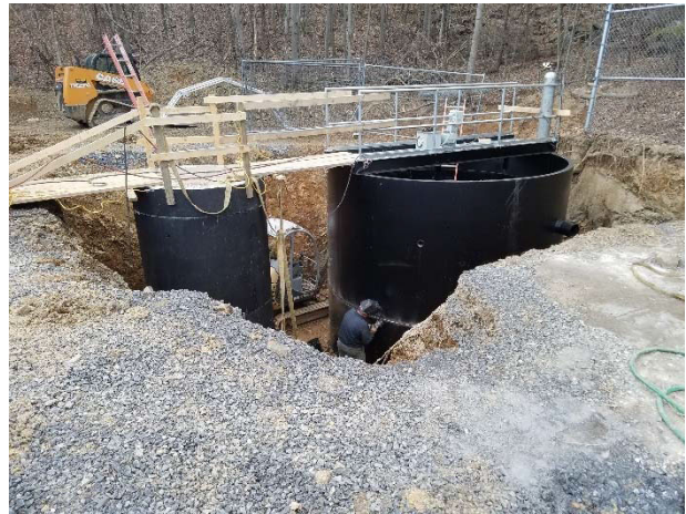
Clarifier and Wet Well Set In Place
