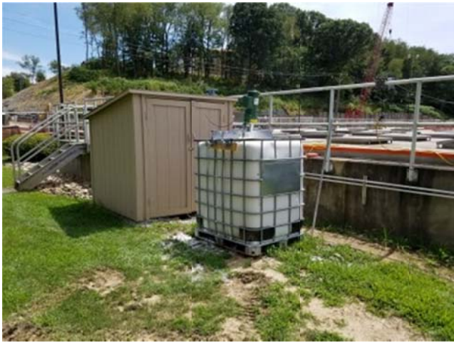
Photo 19: Temporary Magnesium hydroxide addition
