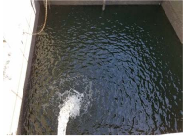
Photo 14: Post-treatment Equalization Tank
