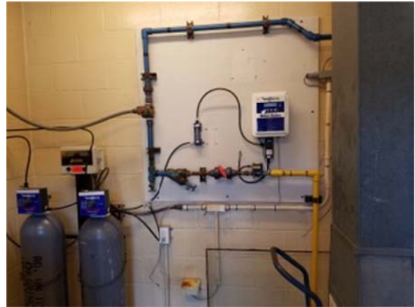
Photo 16: Gas Chlorinator
