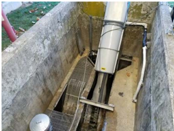
Photo 3: TOC probe at end of Raw WW channel, beside Raptor fine screen and line for NaOH addition
