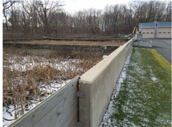
Photo 20: Reed Beds & Solids Loading Station
