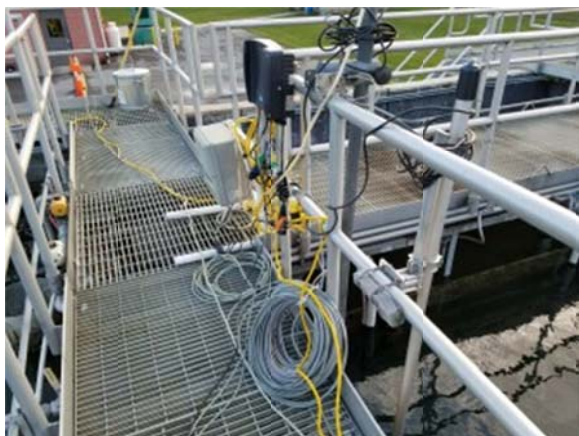
Photo 5: Nutrient immersion probes in clarifier
