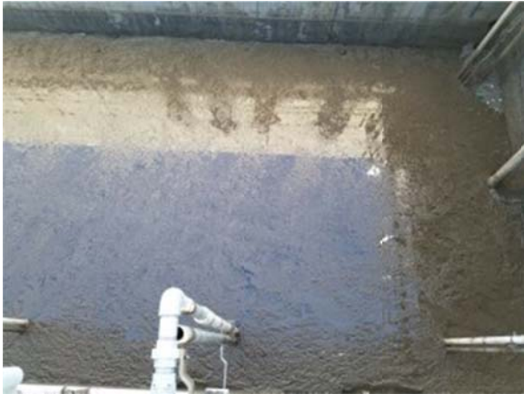
Photo 19: A Digester in Sequox Package Plant
