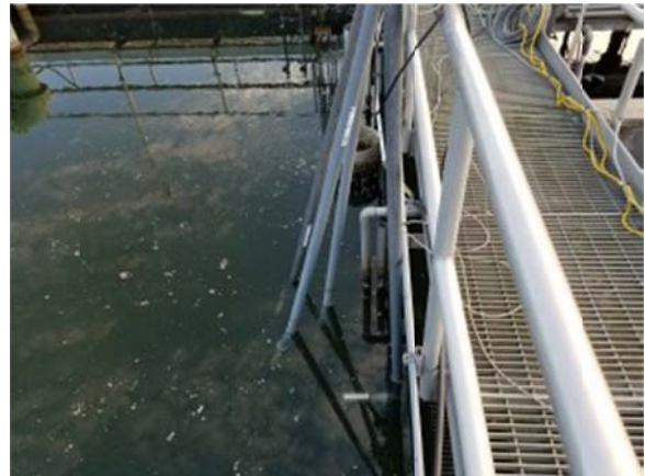
Photo 8: Settling in Tank 1.1 during Off-cycle
