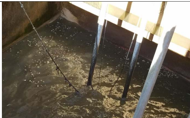
Oil & Grease accumulation in Surge Tank
