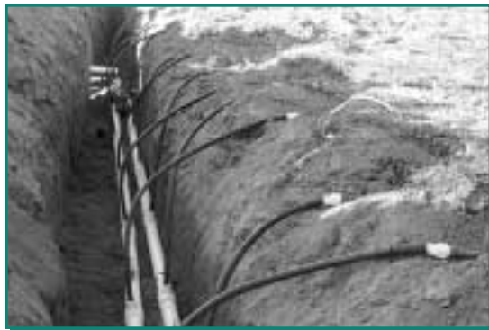
▲ 11. Connecting feed and return lines that supply wastewater to the tubing.
