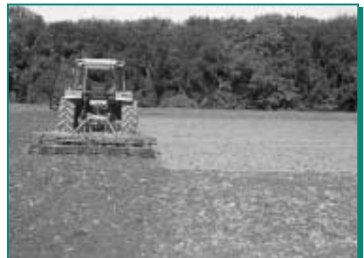
▲ 12. Preparing the soil over the tubing for seeding.
