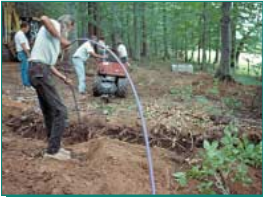
Drip tube installation
