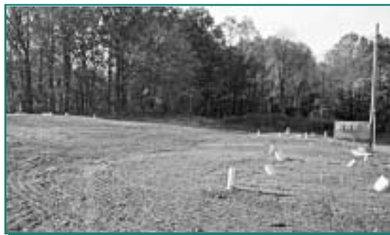
At-grade beds after installation
