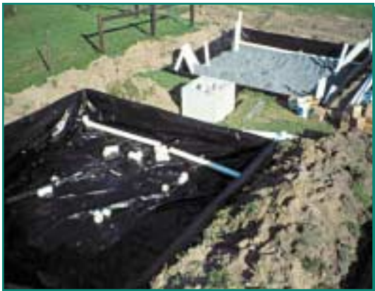
Wetland Cell construction
