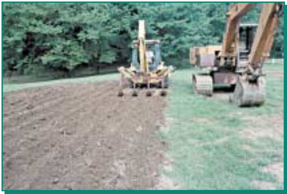
Placement of gravel on at-grade beds
