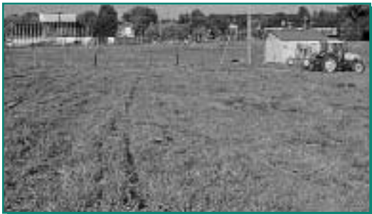
▲ 18. Tubing installed in the pasture.
