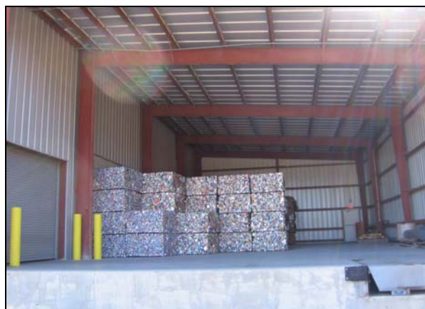
Figure 2-6 Covered Storage Area for Baled Materials
