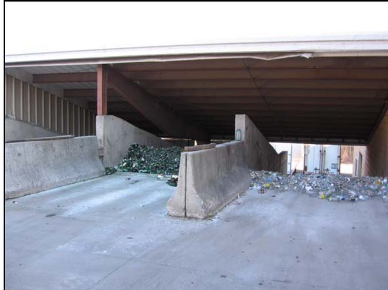
Figure 4-4 Glass Unloading Area
