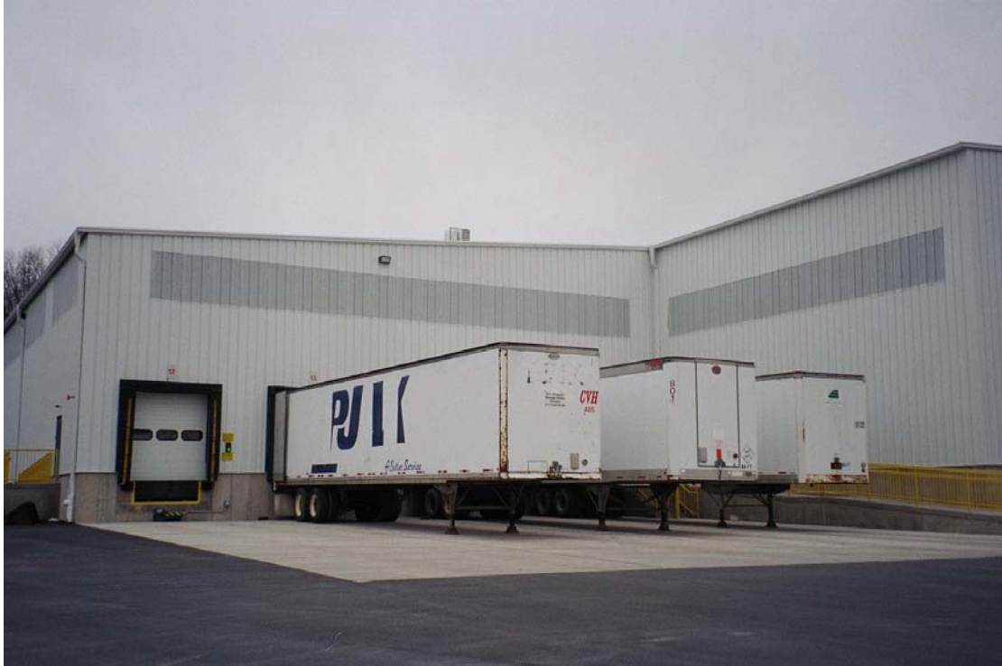
Figure 1 Loading Bays at Lycoming County MRF
