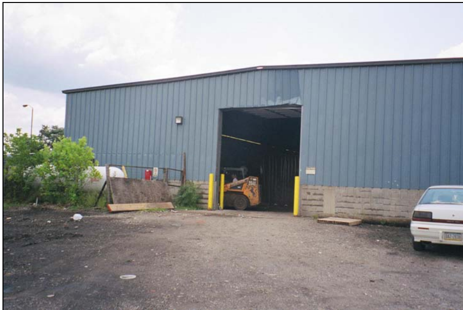
Figure 3 North Entrance to Commingled Container Tip Area
