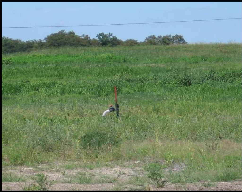
Photo 5: Landfill Gas Well Head
