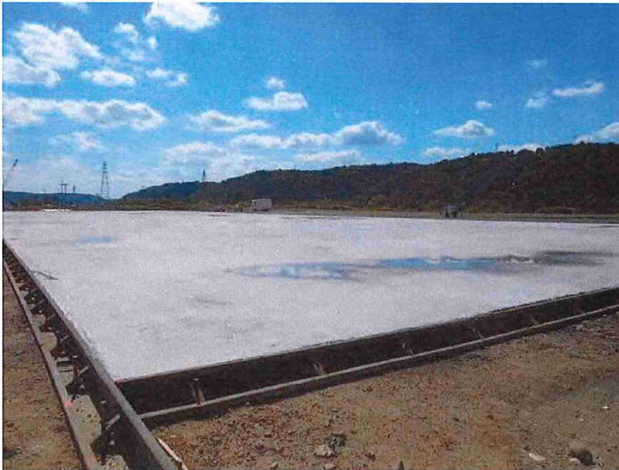
Photo 1 – Typical view of concrete pad installed over No Dig Zones 1, 2, and 3
