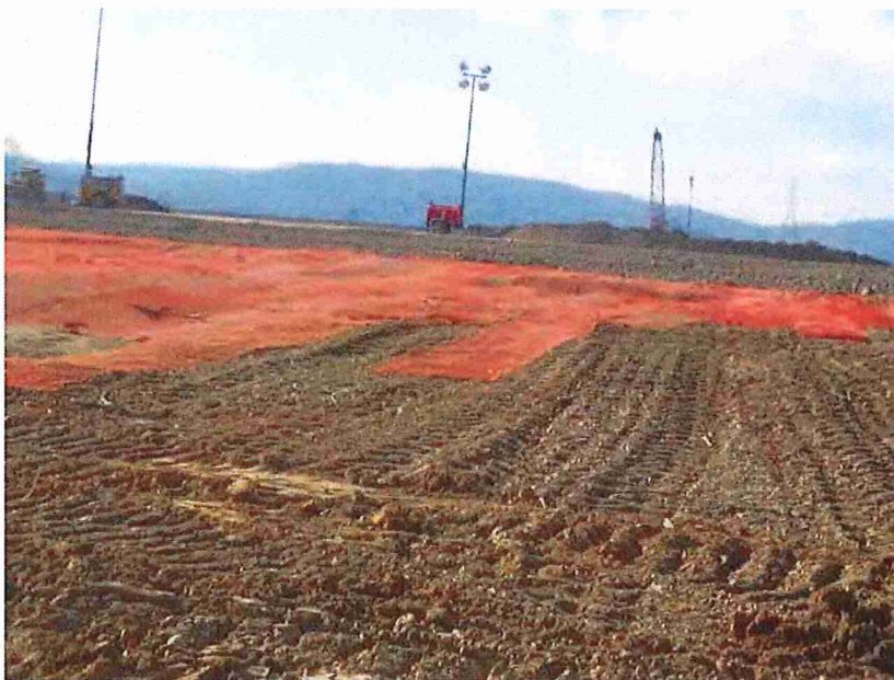
Photo 3. View showing installation of snow fencing and soil placed above geosynthetic liner in soil to groundwater Areas 2 and 3.
