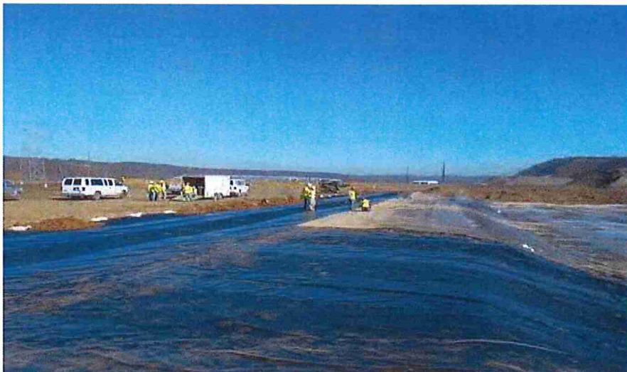
Photo 2. Typical view of geosynthetic liner installed to isolate soil to groundwater concern areas.
