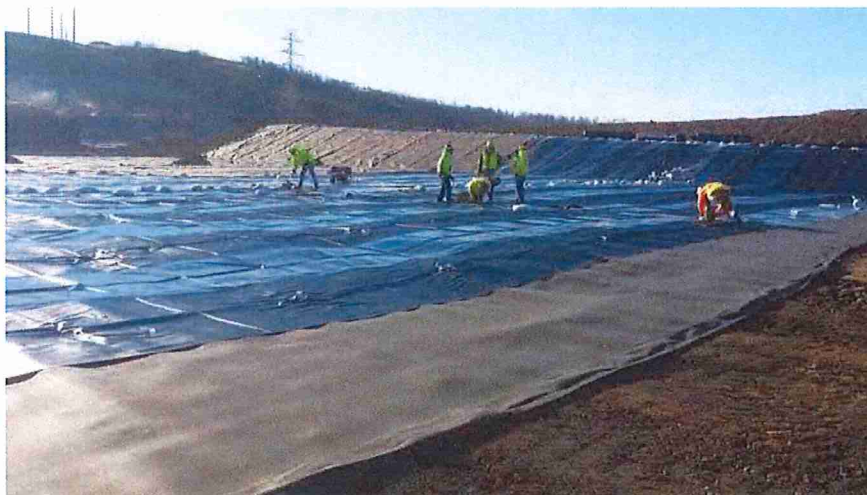
Photo 5. Typical view of the low-permeability liner installed at the Brick Landfill.
