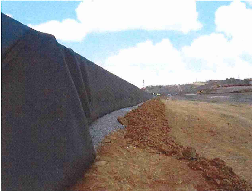
Photo 4. View of the liner placed around the Poorhouse Run box culvert.
