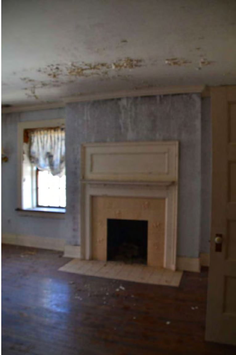
Photo 17: Former Servants Room 1, Second Floor
