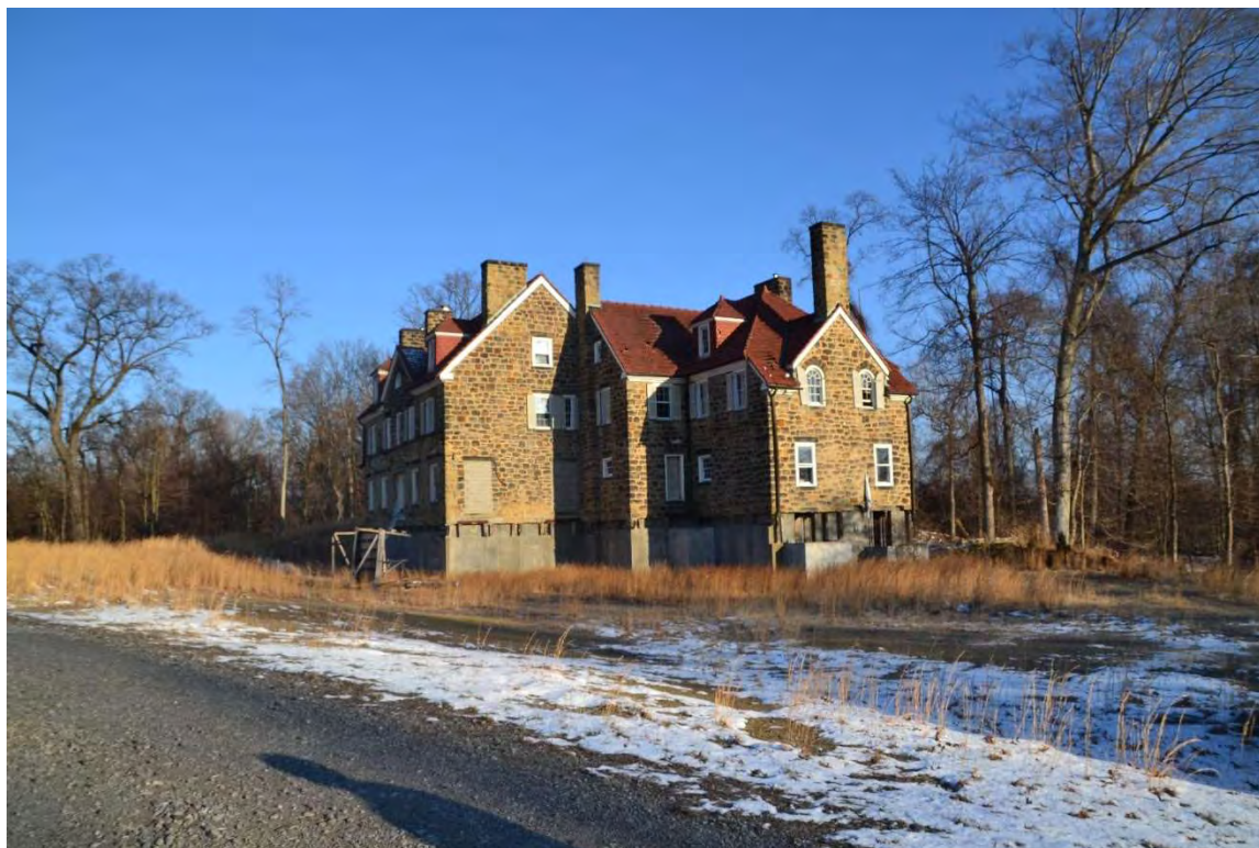
Photo 5: South Side of Residence, Looking North
