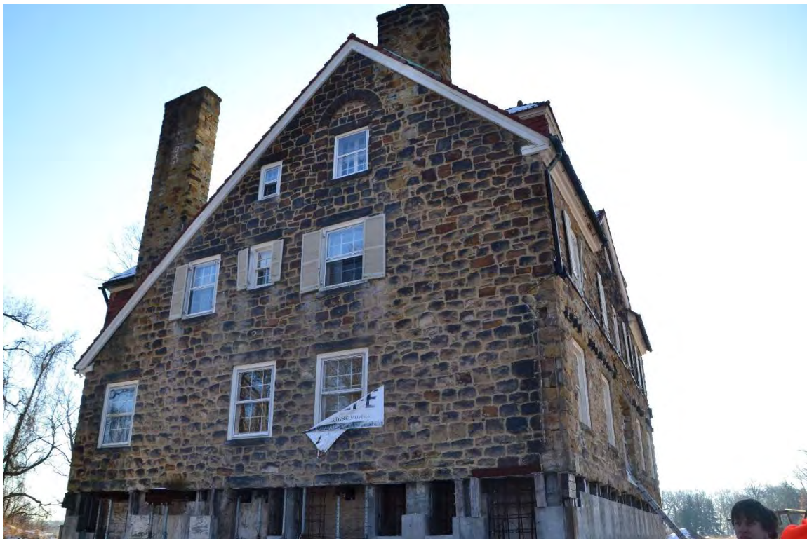
Photo 2: North Side of Residence, Looking South
