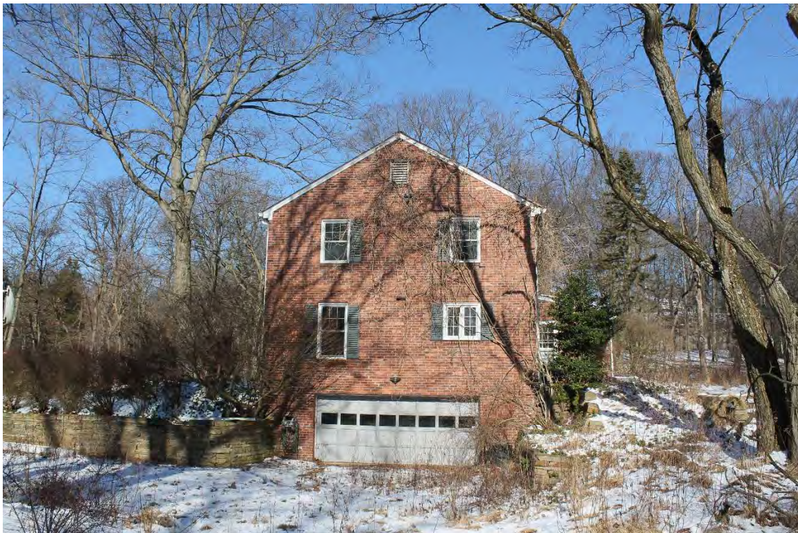
Photo 4: South Side of Residence, Looking North
