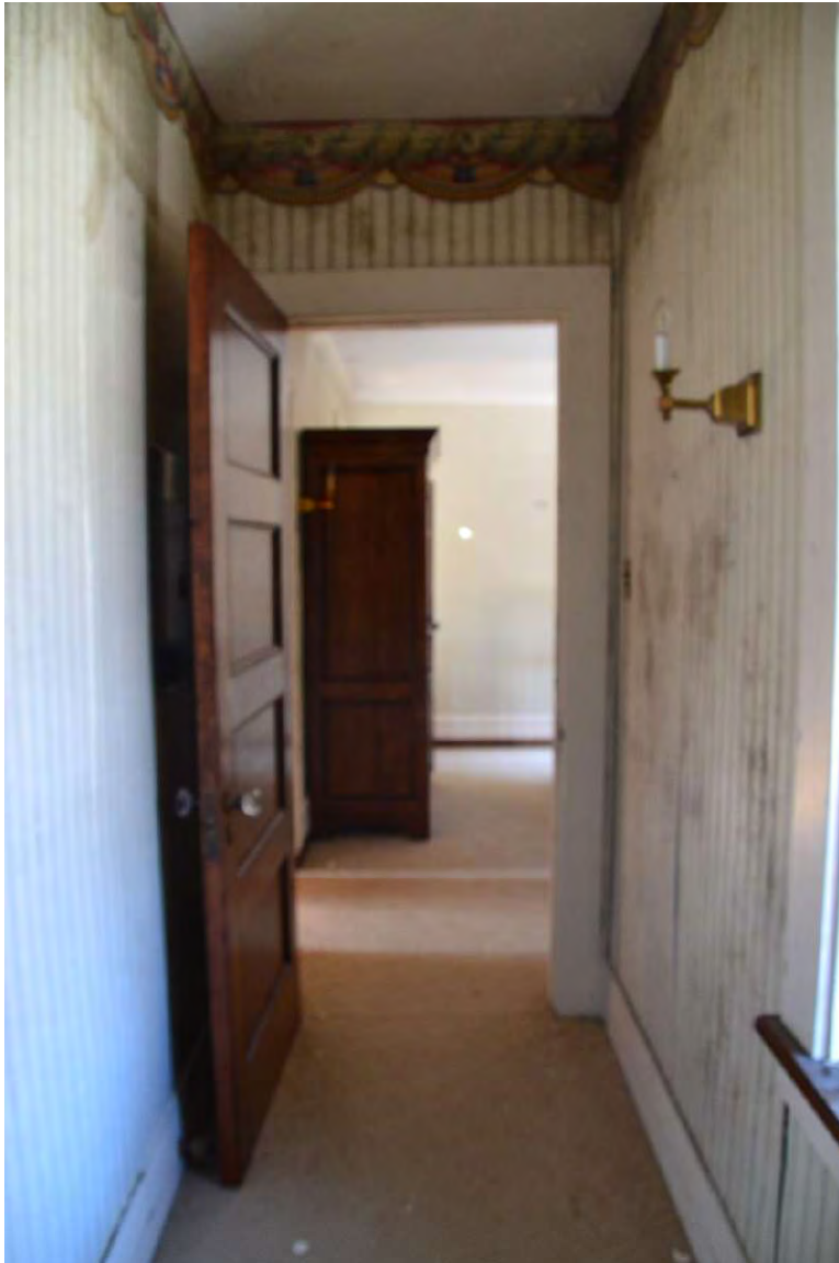
Photo 18: Second Floor Hallway
