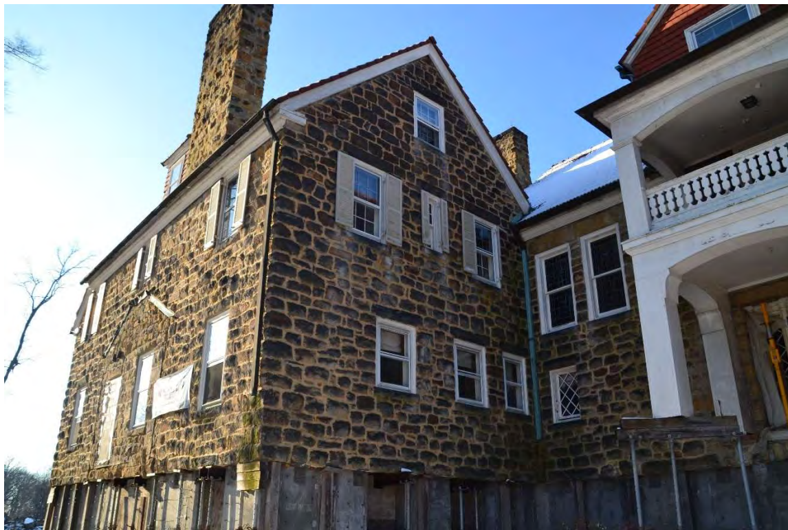
Photo 4: Rear of Residence, Looking South
