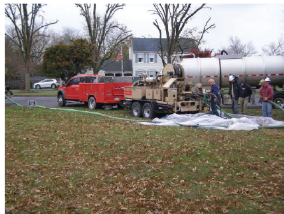
Potable water being used from truck to inject into well 11-10-25
