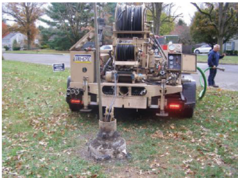
Hydrofracking set up 11-10-25
