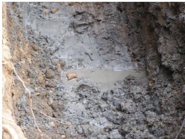
Water in excavation; no visual signs of impacts 9-29-25 @ 12:34
