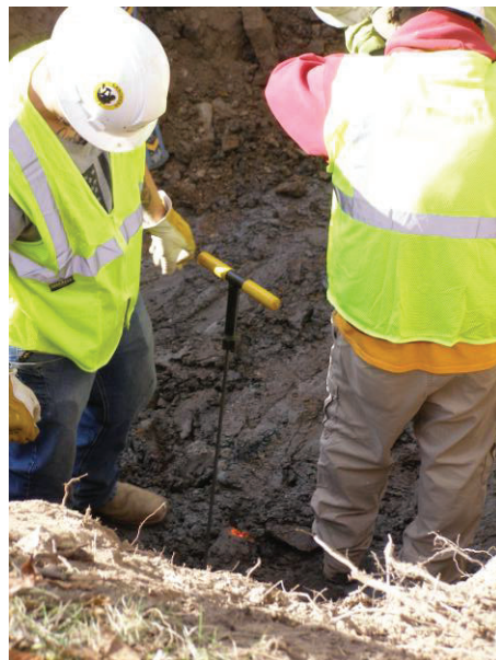
Metal probe used to determine pipeline location 9-29-25 @ 10:14
