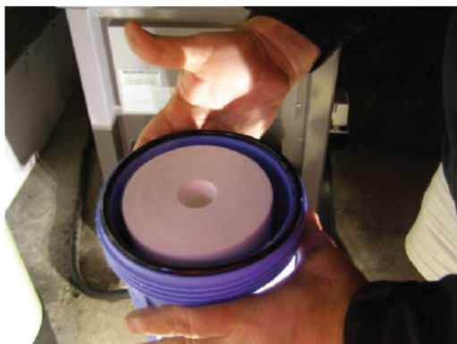
Clean filter - replacement 9-27-25 @ 9:53
