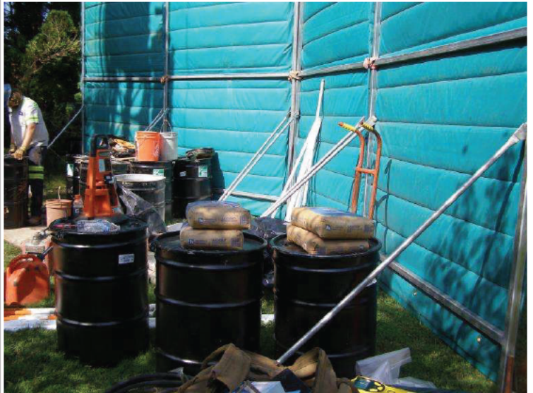
Photo 4: Drum staging and sound barrier
