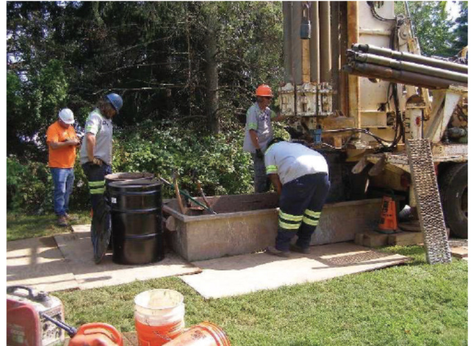
Photo 2: Drill rig placement and set up
