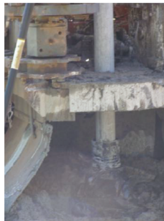
Drill rig setup over well hole after reaching 150 feet bgs. 9-18-25 @ 10:58
