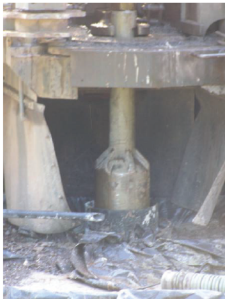
Drill rig set up over grouted well 9-18--25 @ 9:33am
