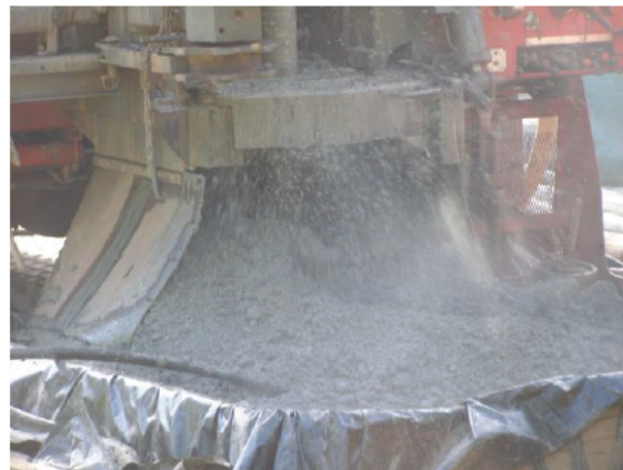
Grout from well while drilling to 81 feet bgs. 9-18-25 @ 9:47
