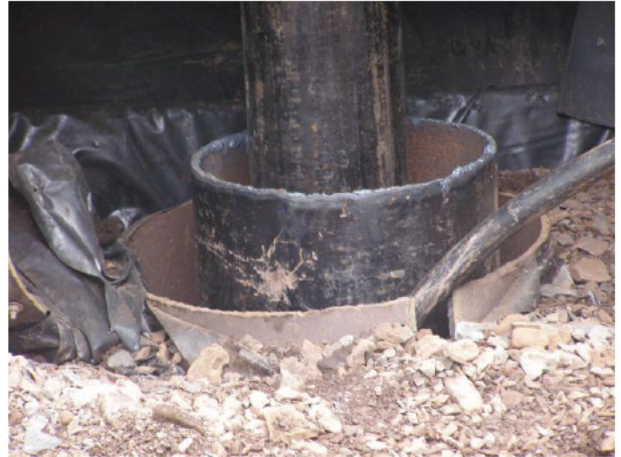
Close up of drill set up at [REDACTED] – side view 9-17-25 @ 9:39
