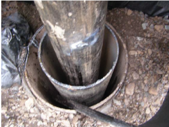
Hose pumping grout into the well – top view 9-17-25 @ 11:55
