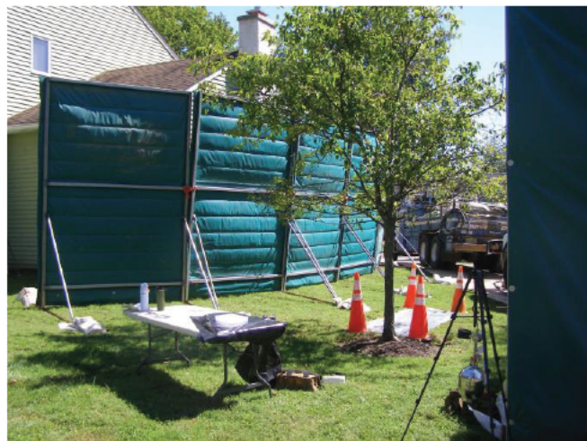
Sound barriers between house and drill rig 9-8-25
