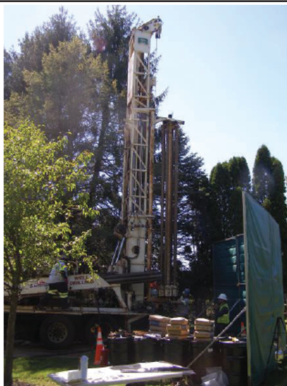
Drill rig set up at [REDACTED] 9-8-25
