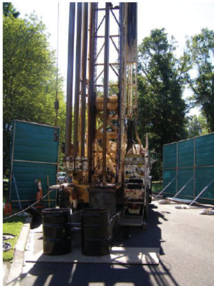
Drill rig set up on Spencer Road at monitoring well location MW-9D 8-26-25 @ 9:39am
