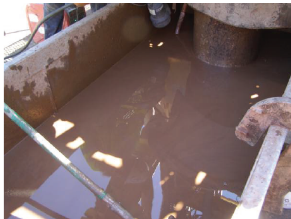
Groundwater from installation of MW-9D that was to be vacuumed 8-26-25 @ 11:13am
