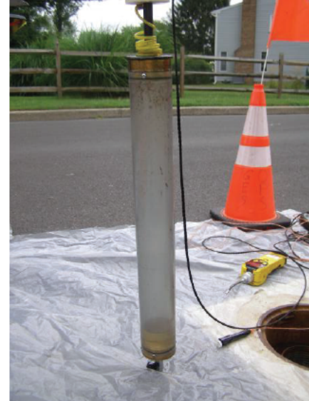
LNAPL in removed skimmer from RW-3 8-25-25 @ 11:11 am
