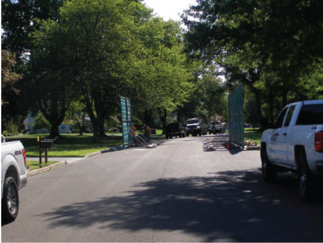
Sound barriers set up on Spencer Road at monitoring wells location MW-9S and MW-9D 8-25-25 @ 9:47am
