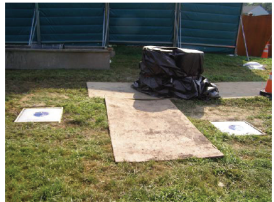
Completed well pads for monitoring wells MW-2S and MW-2D 8-7-25 @ 9:19am
