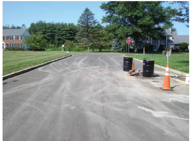
On Spencer Road looking towards Glenwood Drive. Monitoring wells MW-8S and MW-8S on right side of street 8-11-25 @ 10:59am
