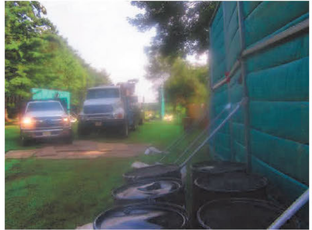
Sound barriers set up – on right hand side looking from cull de sac 7-31-25
