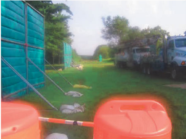
Sound barriers set up – on left hand side from the cull de sac 7-31-25
