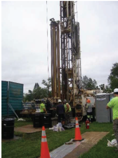
Photo 1: Drilling in progress
