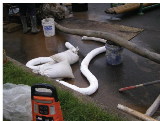
Absorbent booms and pads to soak up sheen along with vacuuming contaminated water from RW-3. 5-22-25 @ 11:26
