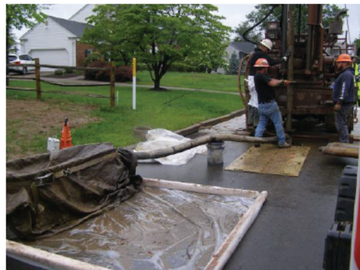
Drill set up for RW-3 on Glenwood Drive 5-22-25 @ 9:46
