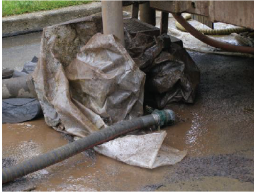
Lewis Vacuum hose in RW-3 to get water before it discharges on Glenwood Drive 5-22-25 @ 11:32
