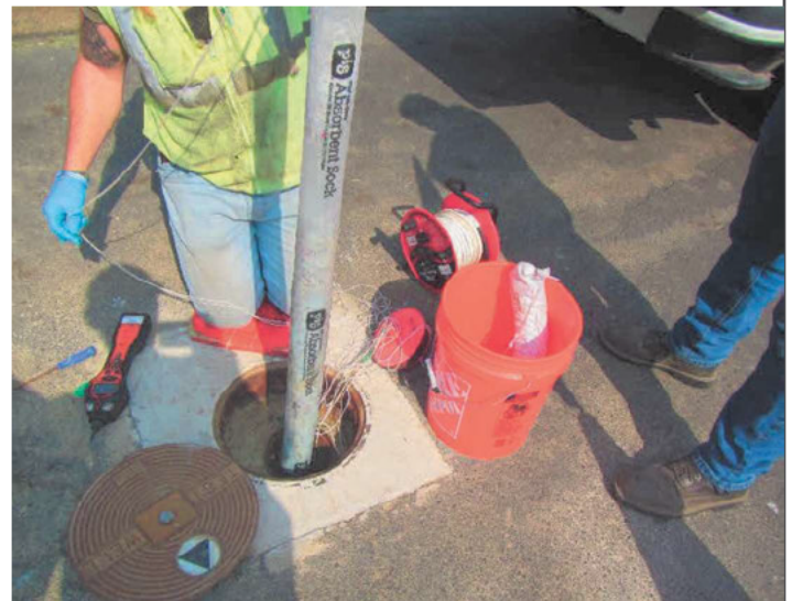
Absorbent sock removal from RW-2.
