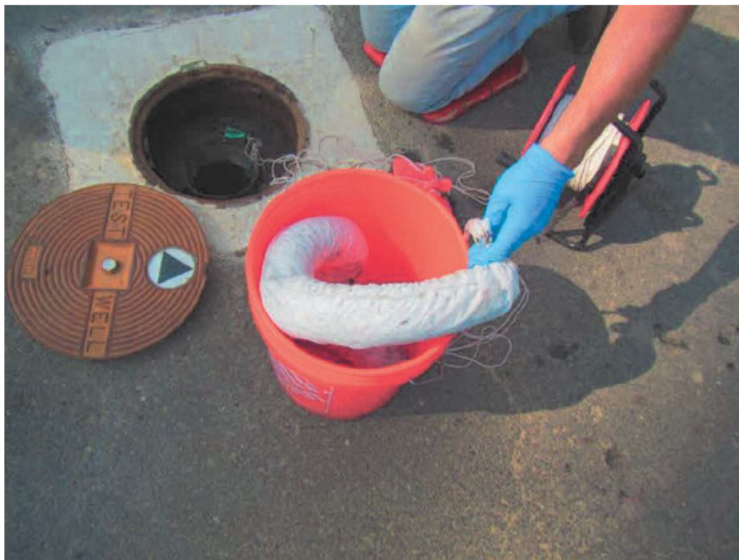
Absorbent sock removal from RW-3.
