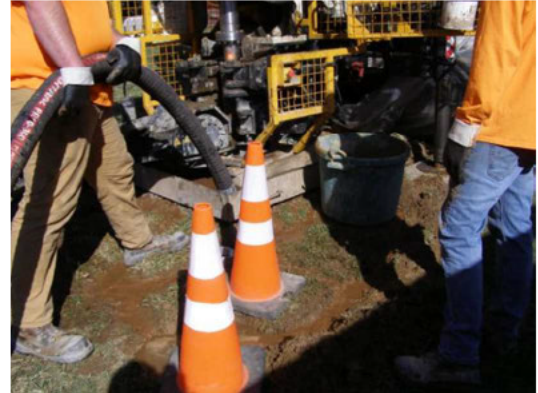
Drill water being vacuumed up at 108 Spencer Road 3-19-25 @ 10:18
