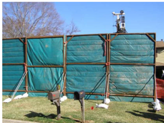
Sound Panels along Spencer Road in front of the drill rig 3/19/25 @ 10:01
