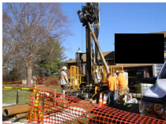
View of drill rig from driveway at 108 Spencer Road 3/19/25 @ 10:02
