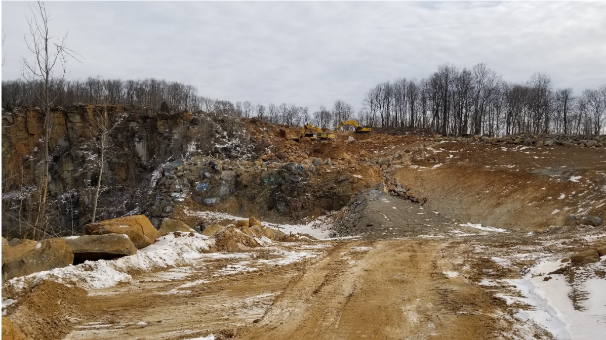
Southern Quarry Working Area
