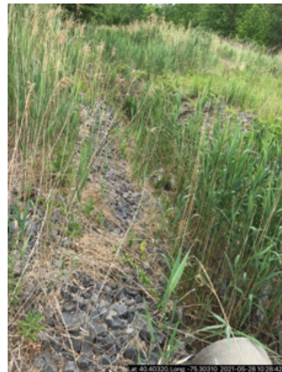
Looking S at outlet of sed trap next to pine trees
