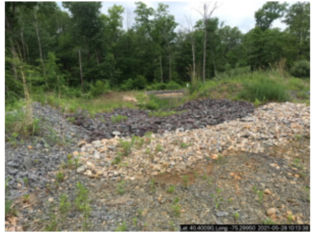
Looking S at inlet for sed trap in S corner
