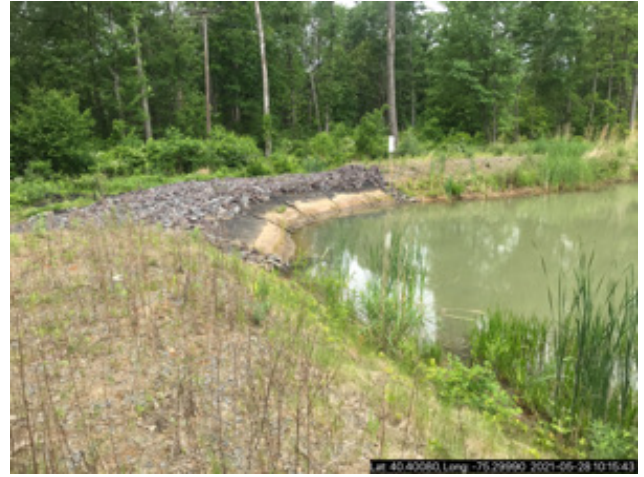
Looking S at emergency spillway
