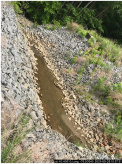
Looking N at last section of discharge channel
