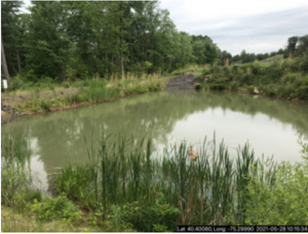
Looking W at water in sed trap
