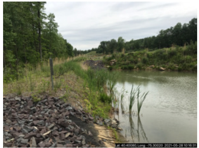
Looking W at second inlet
