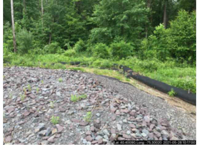
Looking at silt sock along bottom of sed trap
