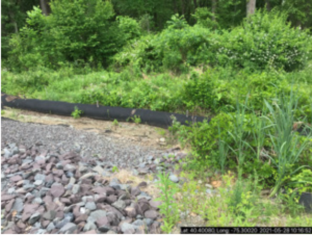
Looking S at silt sock
