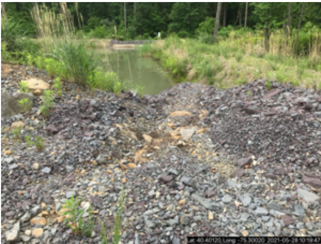
Looking E at second inlet for sed trap
