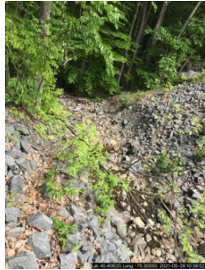
Looking N at outfall
