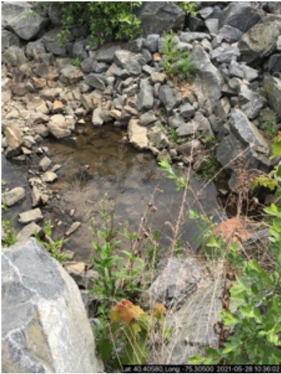
Looking N at inlet pipe to discharge channel
