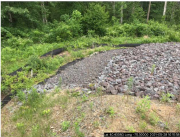
Looking S at area behind sed trap
