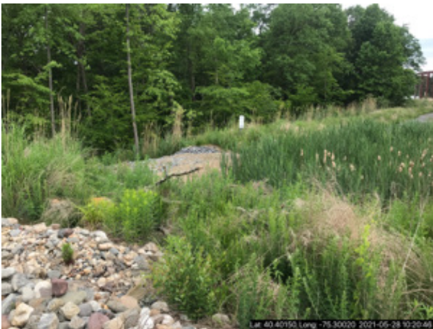
Looking W at emergency spillway for smaller sed trap
