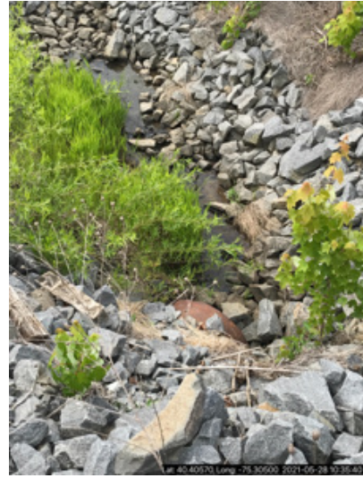
Looking S at inlet to discharge channel
