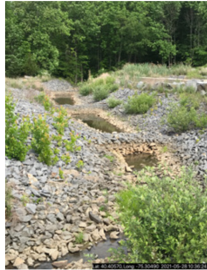
Looking N at discharge channel
