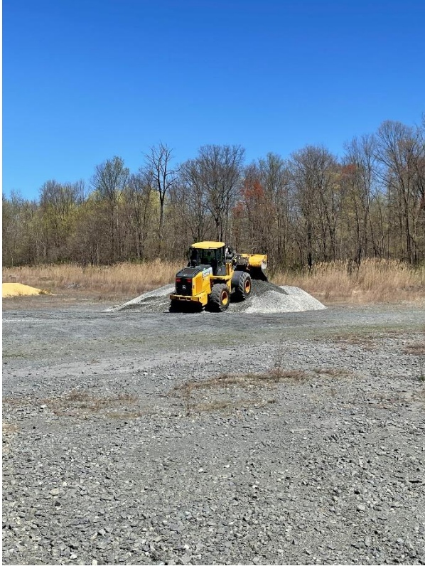
Loader dumping aggregate from wetted stockpile to new stockpile area - 4/12/23, 12:04 PM
