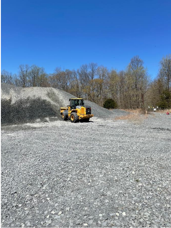
Loader getting aggregate from wetted stockpile - 4/12/23, 12:01 PM
