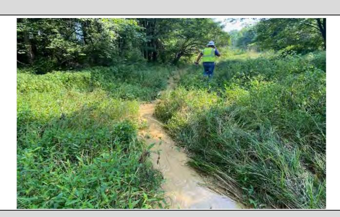
View of drilling fluid within WL-H17 at location of IR release point.
