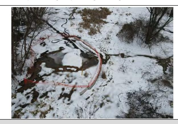
View of earth feature two filled with 28 cubic yards of flowable fill.
