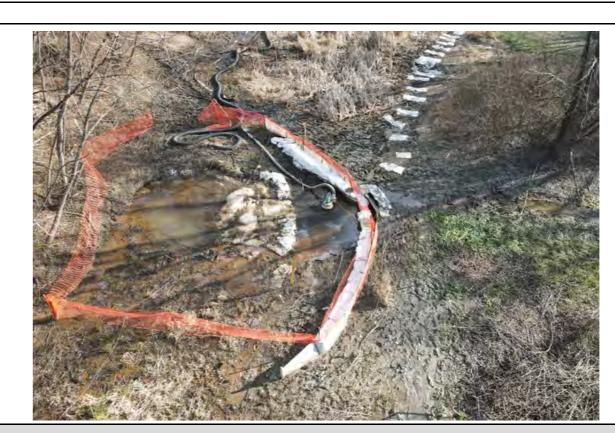
Notes: Notes: View of IR release location and containment within WL-H17. View of contractor crew members installing erosion control blanket to stabilize earth feature locations.
