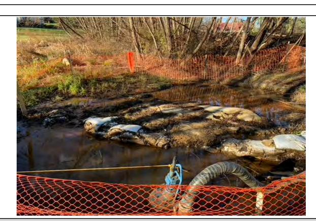
Notes: Notes: View of IR release location and containment within WL-H17. View of IR release location and containment within WL-H17.
