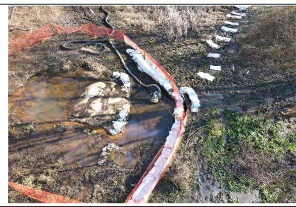
Notes: View of IR release location and containment within WL-H17. View of IR release location and containment within WL-H17.
