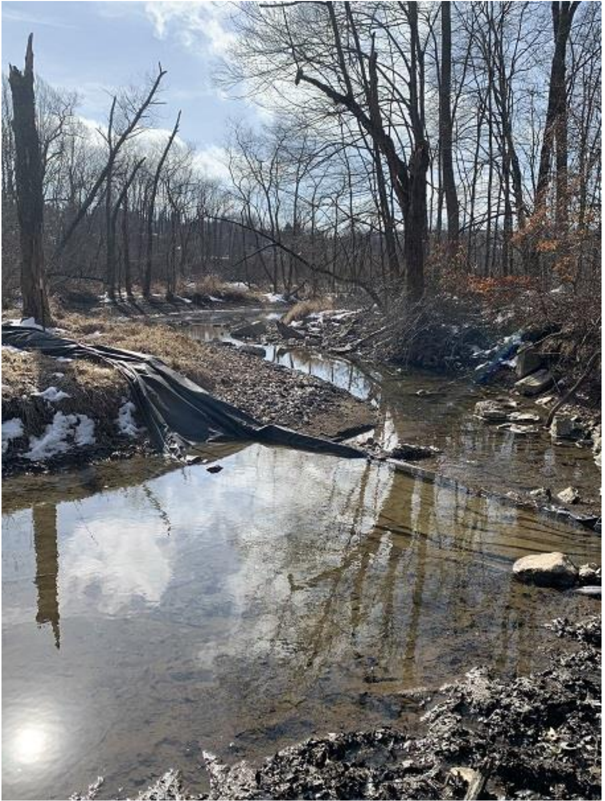
Turbidity Curtain prior to confluence with Ranger Cove
