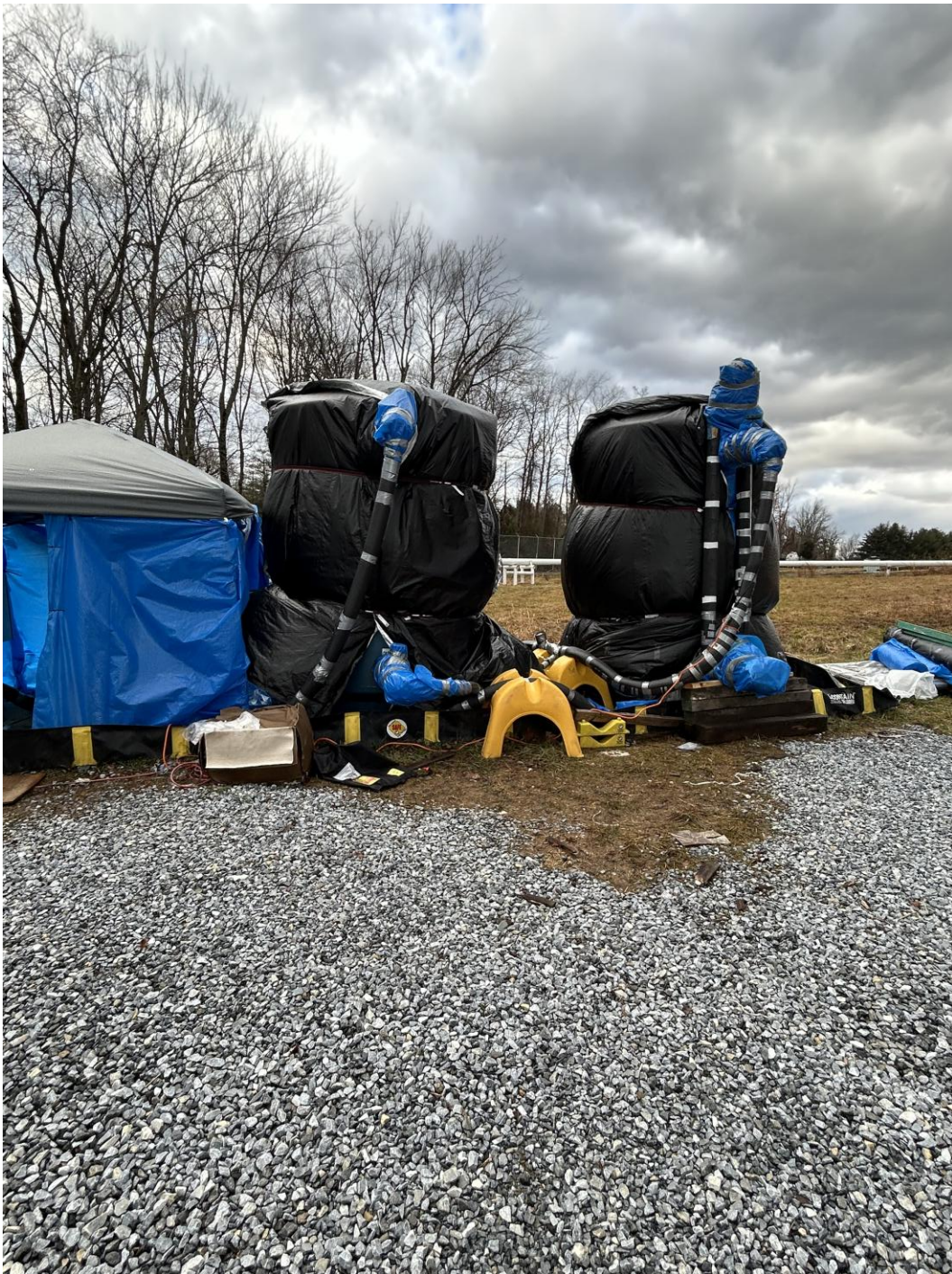
Activated carbon vessels
