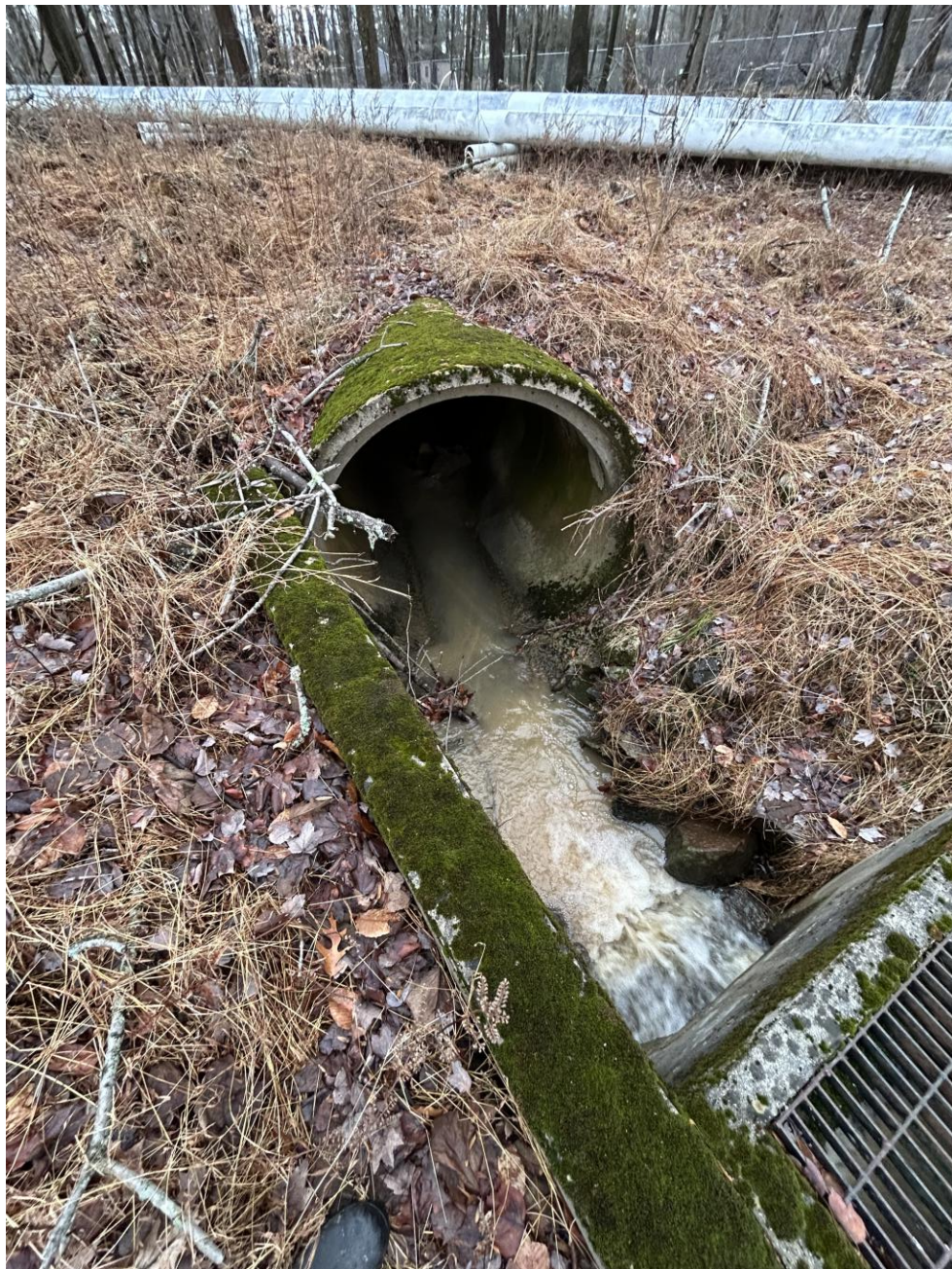
Basin effluent to swale
