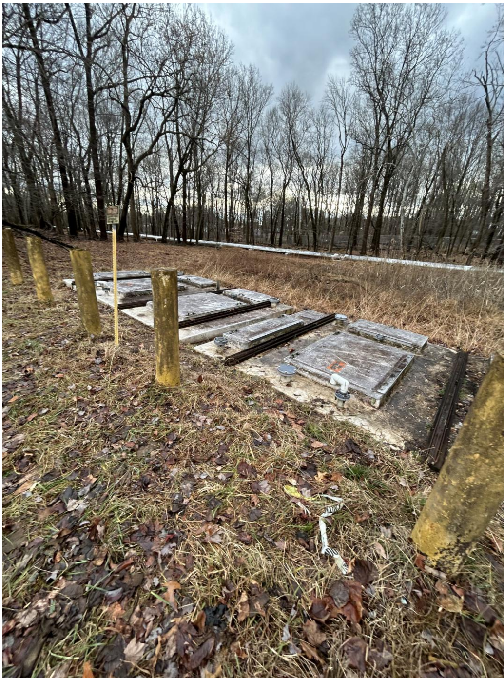
Oil water separator prior to retention basin
